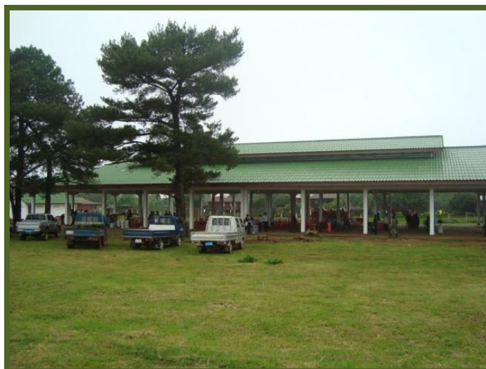
PHOTO 7: CENTRAL MARKET AT PAKXONG DISTRICT
