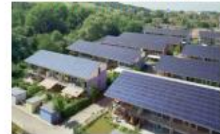
Combined biomass heating and power generation
