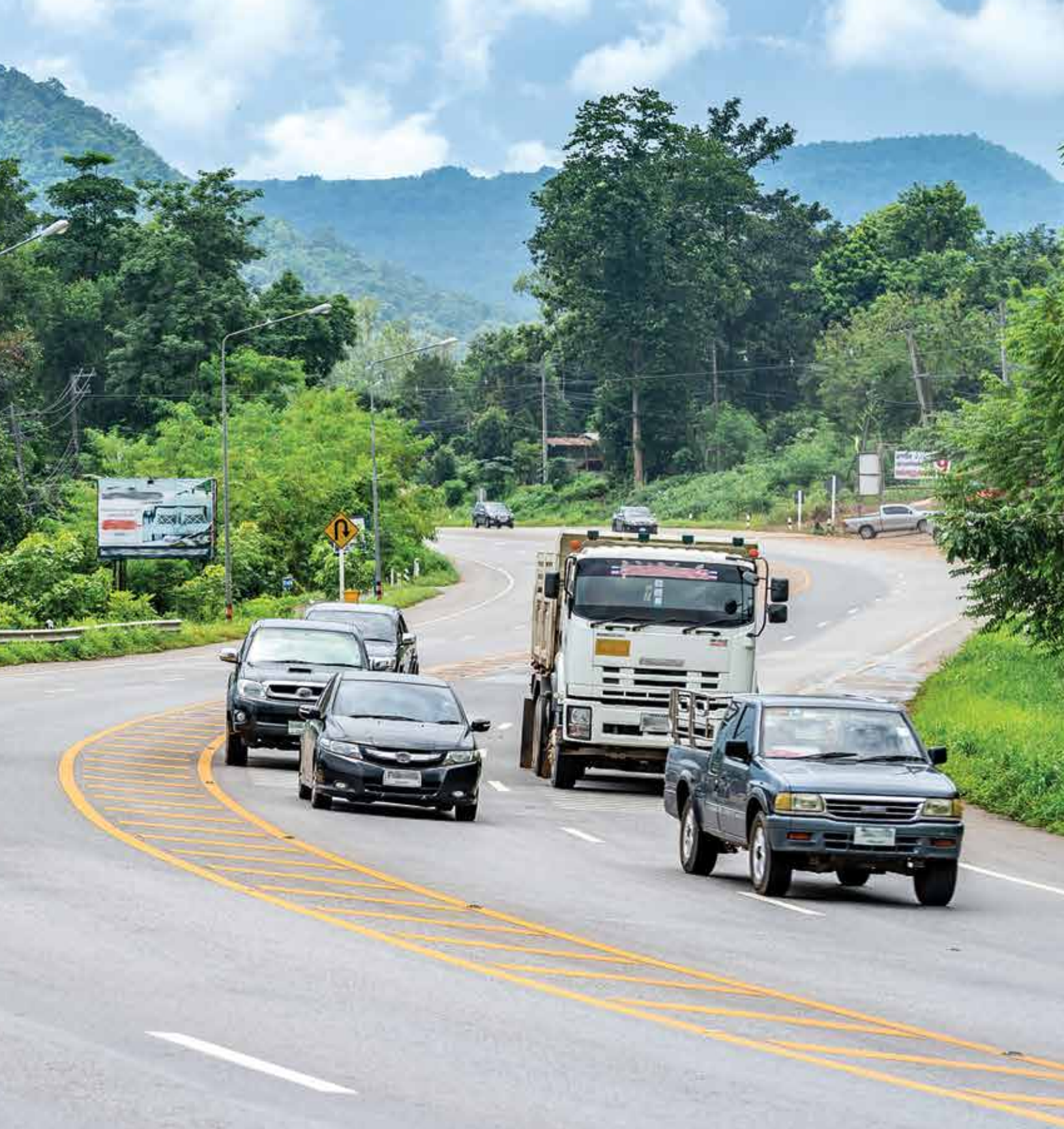
Highway 12 from Phitsanulok to Lom Sak, Thailand (105 km). As a main intersection of the East-West Economic Corridor and the North-South Economic Corridor, the new four-lane highway is a regional gateway creating wider opportunities for cross-border trade, tourism, and investment in Thailand, the Lao People's Democratic Republic, Myanmar, and Viet Nam. The Highway 12 expansion from two lanes to four was supported by Asian Development Bank (photo by Ariel Javellana/ADB).
