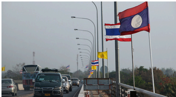
The Thai-Lao Friendship bridge built with Australian funding, crossing the Mekong River. Photo by Australia DFAT (CC BY 2.0).
