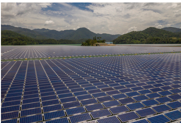
Aerial view over the floating solar photovoltaic (PV) power generation panels at the Da Mi hydro power plant in Viet Nam.
