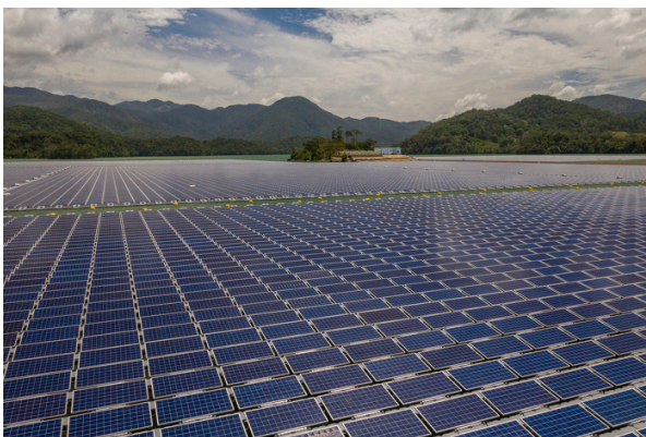
Aerial view over the floating solar photovoltaic (PV) power generation panels at the Da Mi hydro power plant in Viet Nam.
