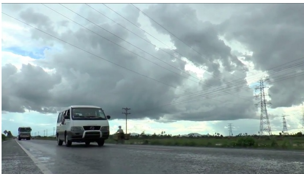
An improved national road in Southern Cambodia.
