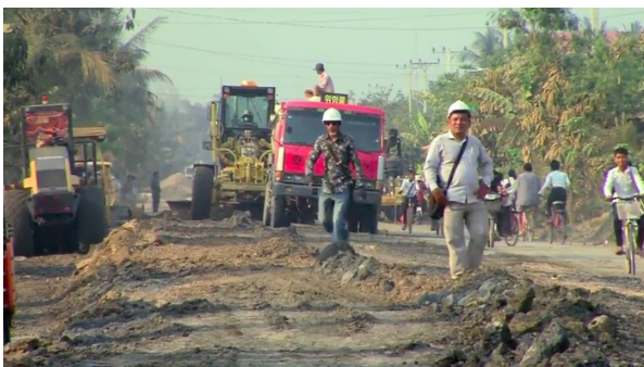
During the civil works of Cambodia Road Improvement.
