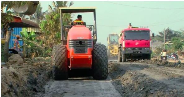
During the civil works of Cambodia Road Improvement.
