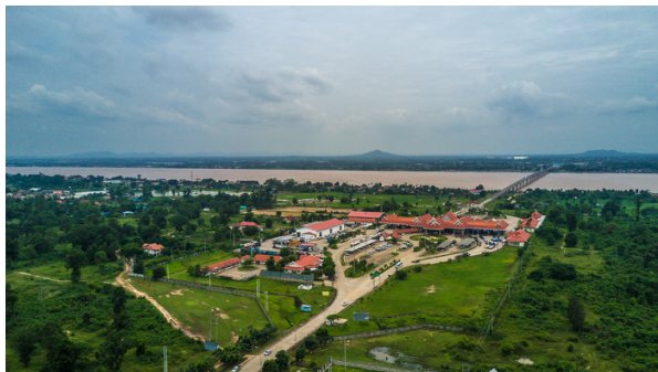
Aerial view of the border check point on the Lao side of the Mekong River. On the horizon is the second Thai-Lao Friendship Bridge which connects Mukdahan Province in Thailand with Savannakhet in Lao PDR.
