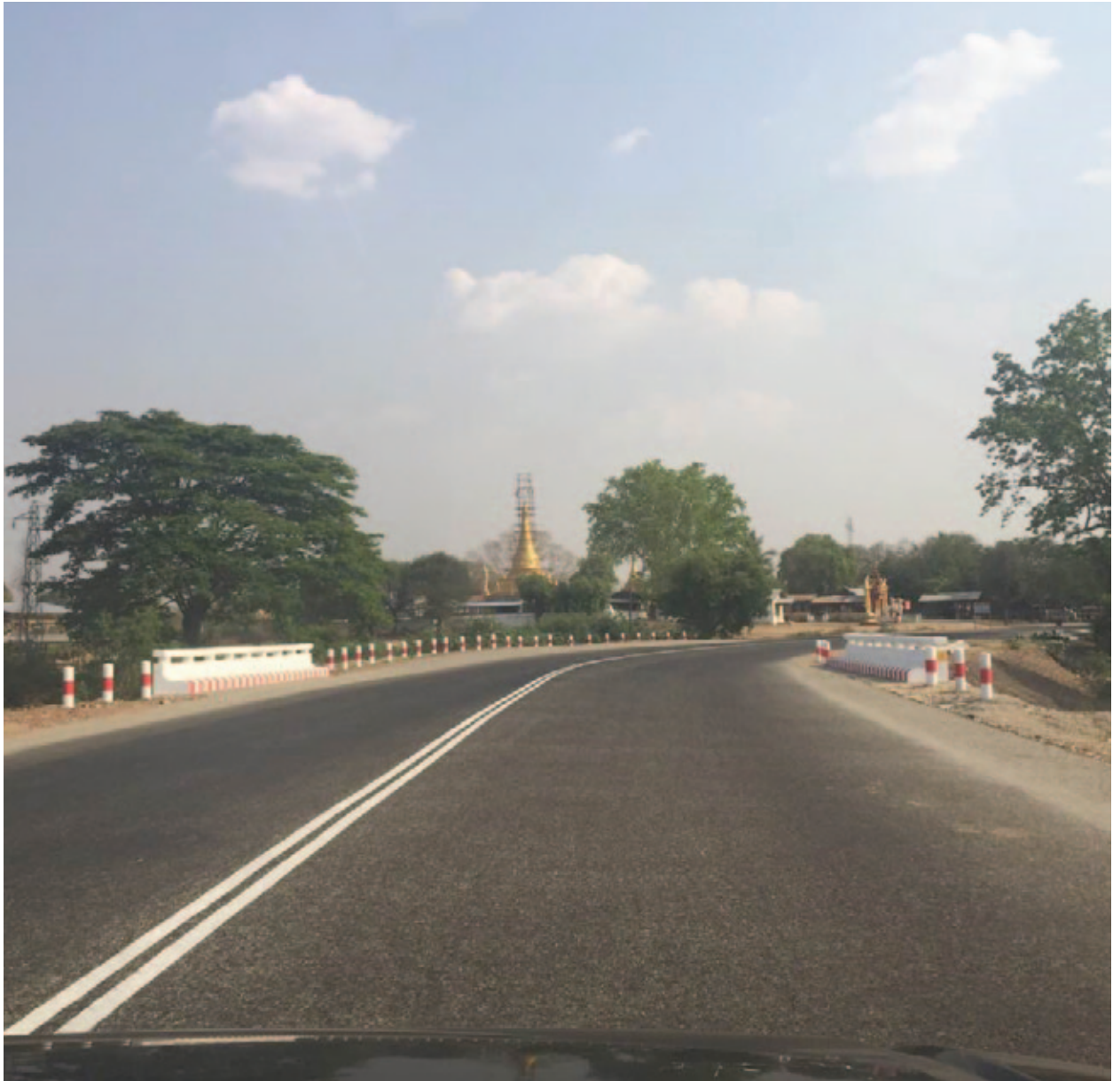
New four-lane road along Yamethin–Meikhtila road section. Yuzana Co. constructed the road by build–operate–transfer.
