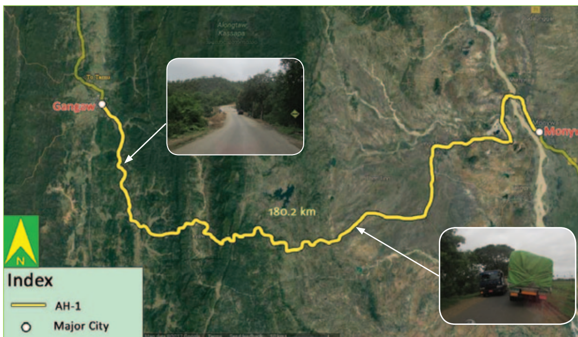
Figure 36: Gangaw–Monywa Road Section
