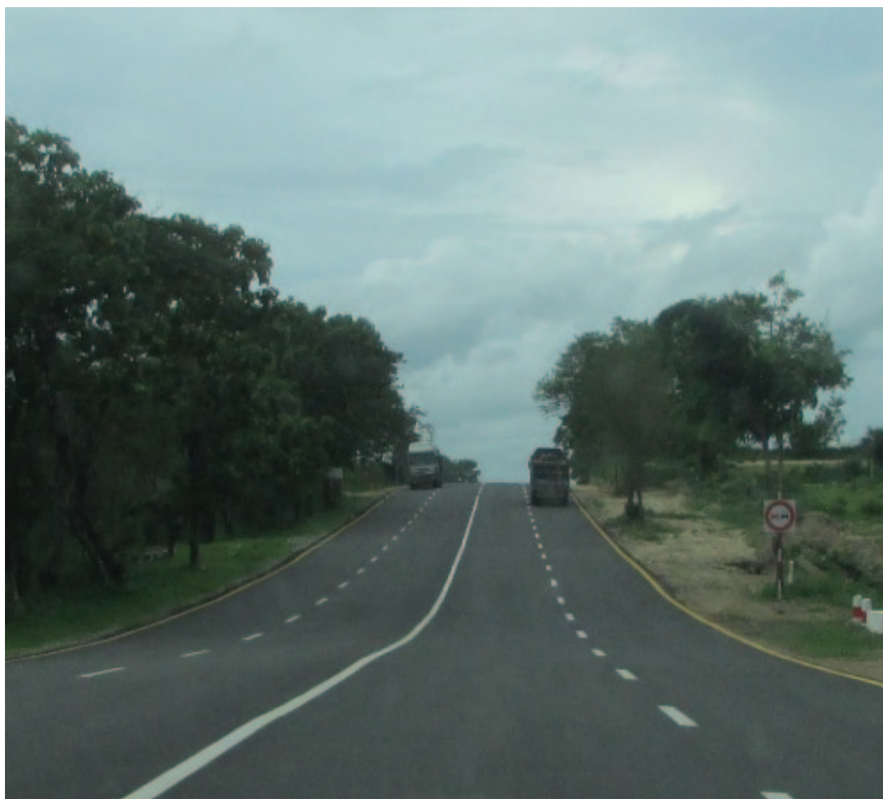
New four-lane road along Nay Pyi Taw–Yamethin road section. Oriental Highway Co. constructed the road by build–operate–transfer; it was opened on 1 July 2017.
