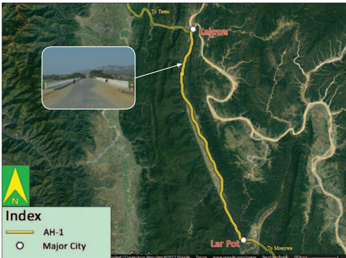
Figure 31: Lar Poh–Kalewa Road Section
