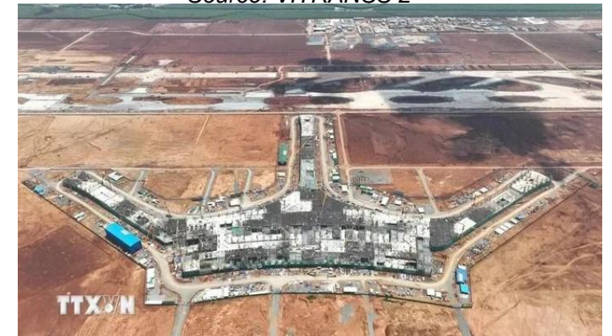
Long Thanh International Airport
